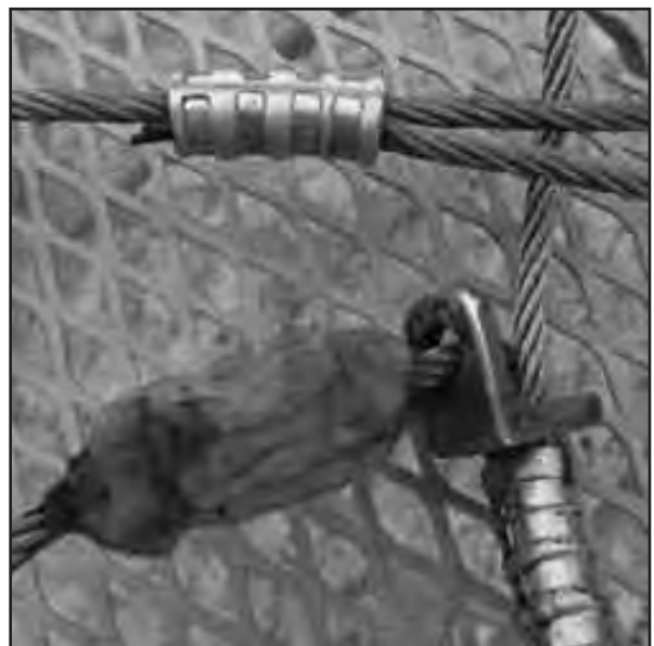
Applied Nycopress clamp covered with silicon glue
